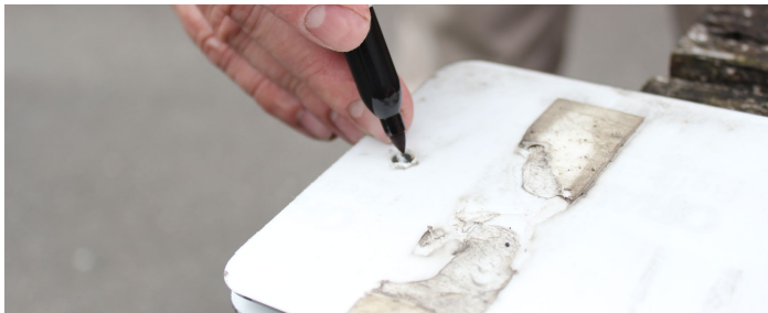
1. Remove existing plate and establish appropriate fixing points.
