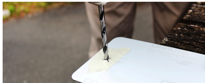
3. Using a 6mm diameter acrylic bit, drill from the REAR of plate. (Allow drill to do the work - don't apply too much pressure).
