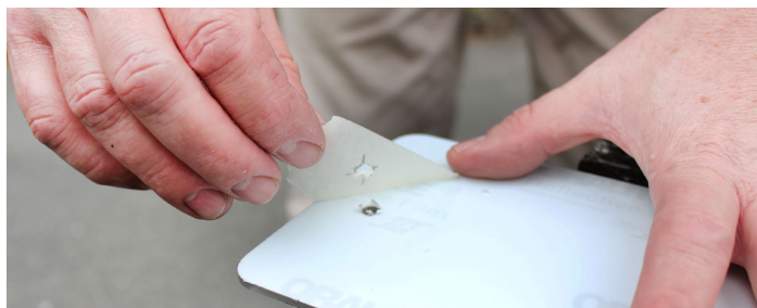
4. Remove masking tape and de-burr holes.
